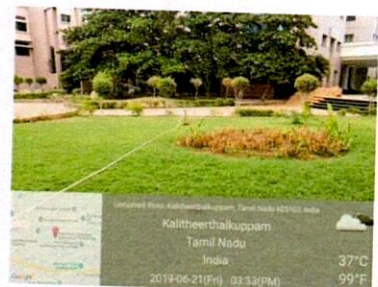
Waste water recycling
